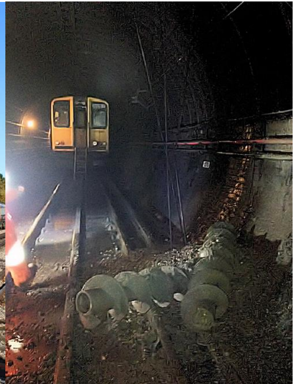
Tube tunnel penetration, London, 2013. Source: RAIB, 2014.
