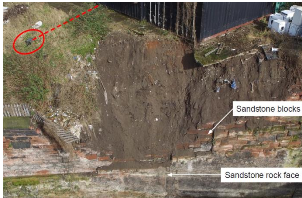
Retaining wall collapse, Liverpool 2016. Source: RAIB, 2017b.
