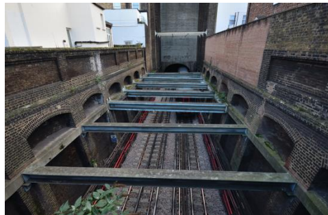
Retaining & Parapet walls; Props
