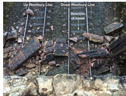
Fallen bridge parapet at Froxfield, 2015. Source: RAIB, 2016
