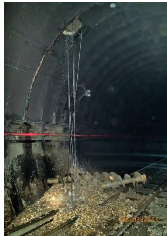
Tube tunnel penetration, London, 2013. Source: RAIB, 2014.
