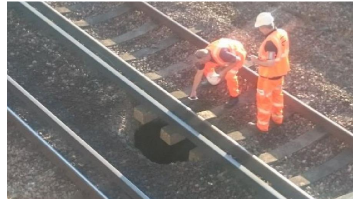
Sewer collapse, Forest Hill, 2016. Source: BBC, 2016.
