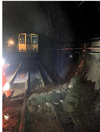
Augers within a tube railway tunnel after penetration, London, 2013. Source: RAIB, 2014.
