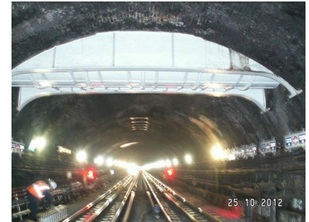
Sewer passing through a sub-surface railway tunnel, London, UK. Source: London Underground.
