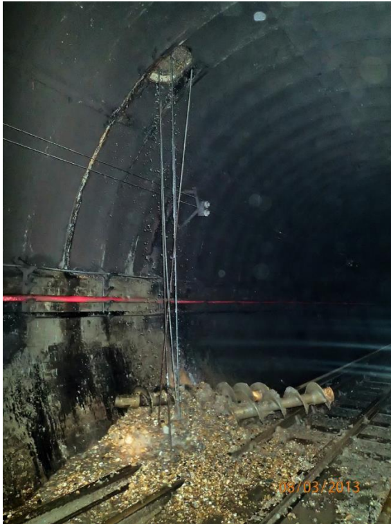
Penetration of tunnel lining and debris on track. Source: RAIB, 2014.
